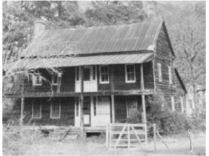
The A. G. Metts House (above) is a two-story structure that features an interior rear chimney in addition to an exterior one. The house was built in 1900 and moved to its present site near 1941 as Lake Moultrie flooded the area.
