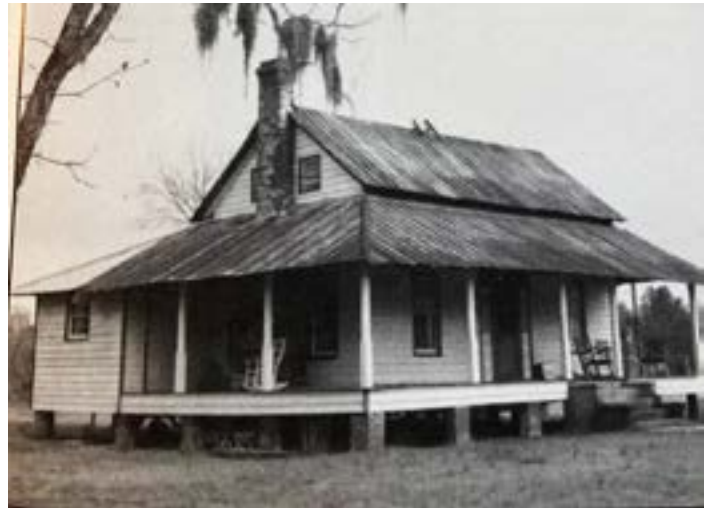
The John M. Metts House (above), built in 1900, is another variation of the local theme with one and a half stories and roofed porches on all sides.
