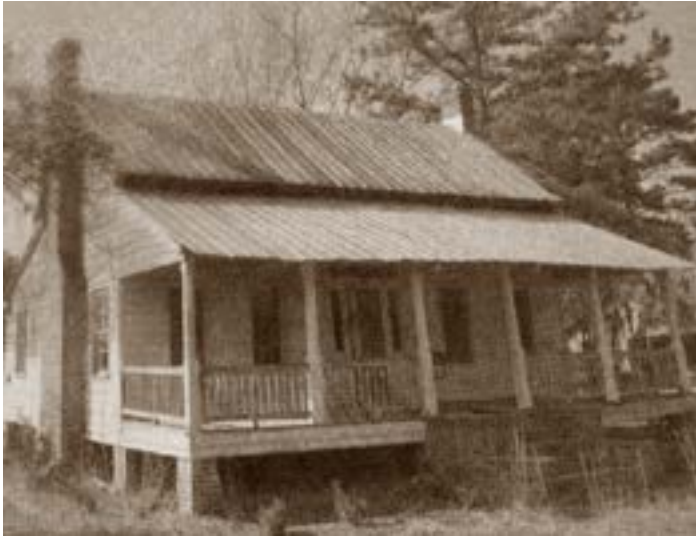
The Robert C. Austin House (above) was built in 1900. It features a gable roof and an exterior end chimney.
