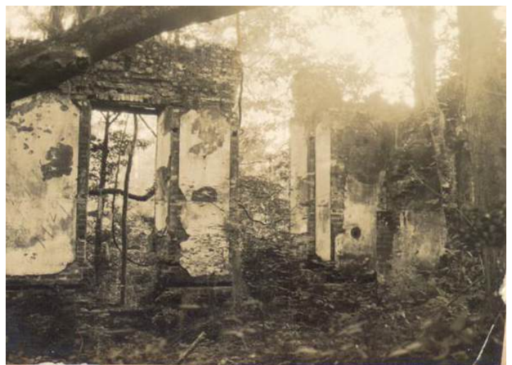
The 1928 photograph shows some of the stucco masonry that smoothed and protected the interior walls. The image also shows a tall airy window openings designed to capture breezes. The photograph is among the William Henry Johnson Scrapbook collection at the South Carolina Historical Society, Charleston, South Carolina.
